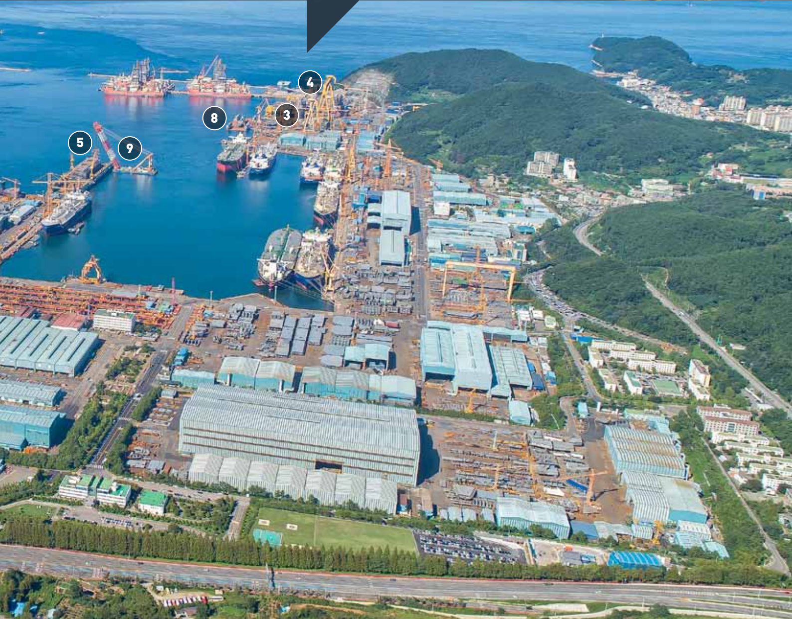
Offshore & Plants Fabrication Area (Heavy Zone)
