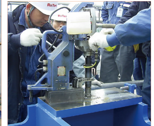
Centrifugal Compressor Bolt Hole Working
