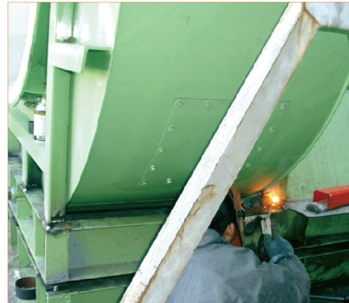
Casing Change of Equipment
